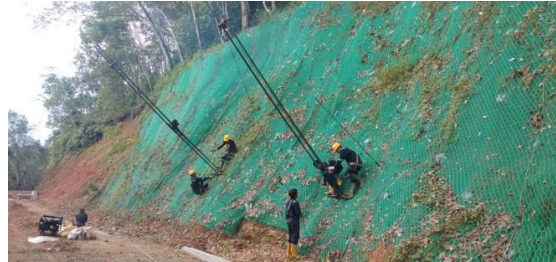
Sinamar Dam, West Sumatra, Indonesia (2020)
