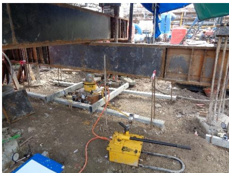
Pile Compression Test – RDMP Balikpapan, Kalimantan Timur, Indonesia (2021)
