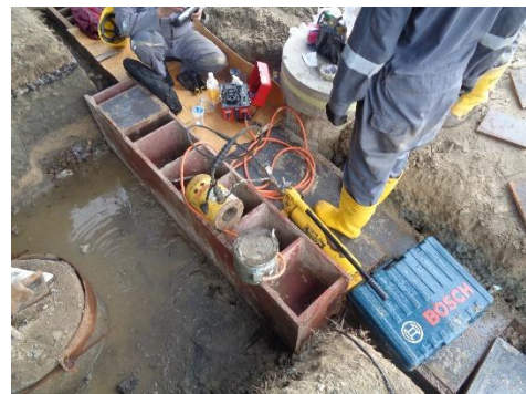
Pile Lateral Test – RDMP Balikpapan, Kalimantan Timur, Indonesia (2021)
