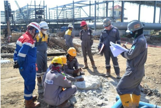
Pengetesan Pile di RDMP Balikpapan, Kalimantan Timur,, Indonesia (2023)
