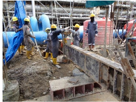
Pile Tension Test – RDMP Balikpapan, Kalimantan Timur, Indonesia (2021)
