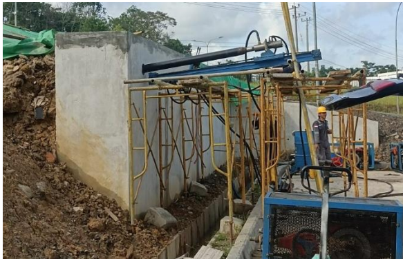
Pemasangan soil nailing di dinding penahan di Kariangau, Kalimantan Timur, Indonesia (2024)
