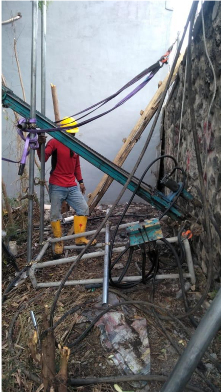
Soil Nailing and Rock Anchor Rig on the Ground
