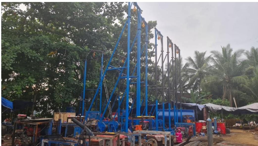
Gate Drilling Rig for Mini Bore Pile and Micropile
